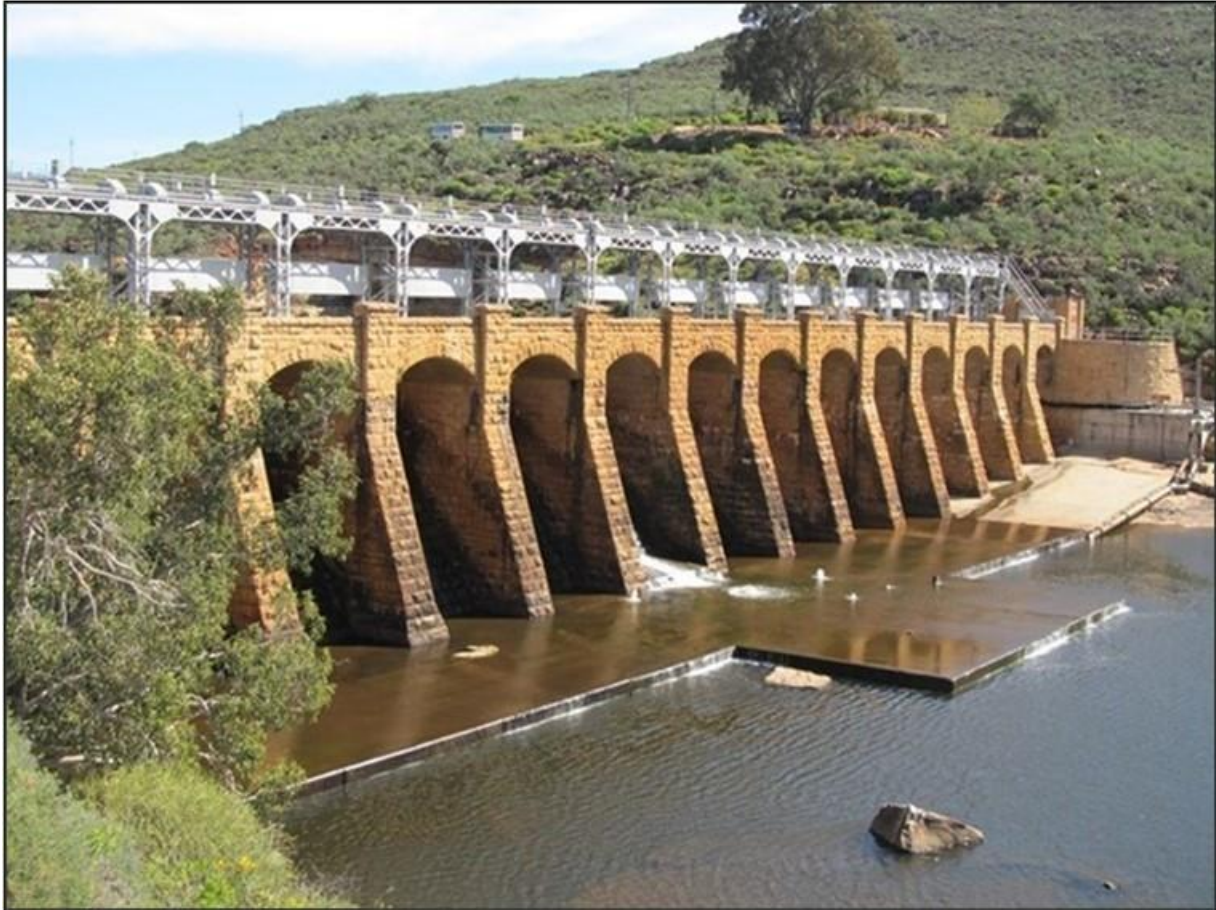
Figure 13-3: Concrete masonry Bulshoek Weir
