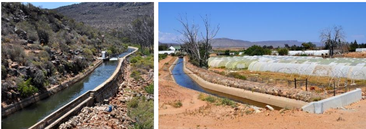
Figure 2-1: The Lower Olifants Canal near Bulshoek Weir (left) and downstream
