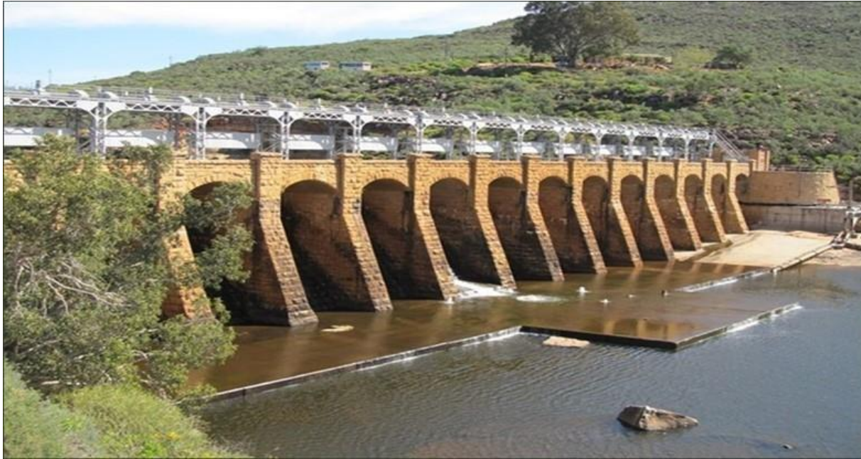
Figure 2-2: Bulshoek Weir on the lower Olifants River
