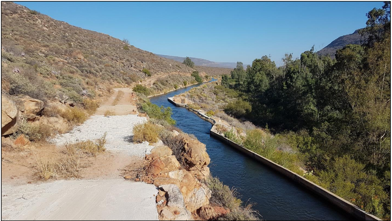
Figure 13-8: Existing Left Bank Canal looking downstream (approx. ch 1.2 km)
